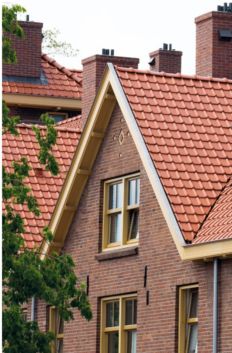
All concrete roof tiles were replaced with ceramic tiles.
